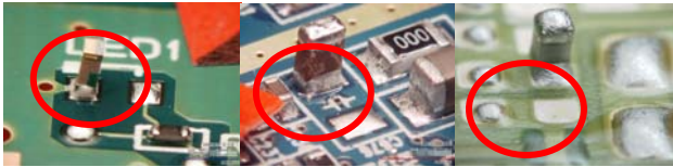
Figure 17: Uplifted capacitors due to varying factors.
