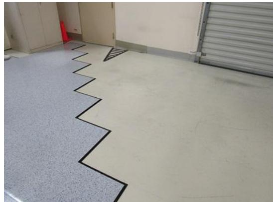
Engineered with a durable conductive polyurethane finish, FreeStyle ESD™ Classic X provides consistent, long-term static control performance along with chemical resistance and simple maintenance. The tiles are available in both conductive and static dissipative options, meet ANSI/ESD S20.20 standards, and are backed by a lifetime electrical warranty and a 10-year limited wear warranty.
