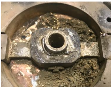
Figure 16. Relatively high amount of dross after two weeks (no maintenance).
