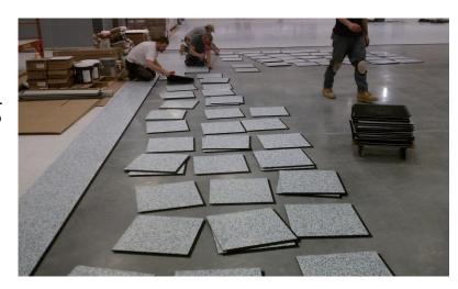
StaticStop conductive and dissipative flooring comes in 18.5 x 18.5"
